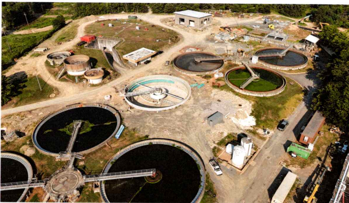
Settling Basin Under Construction
