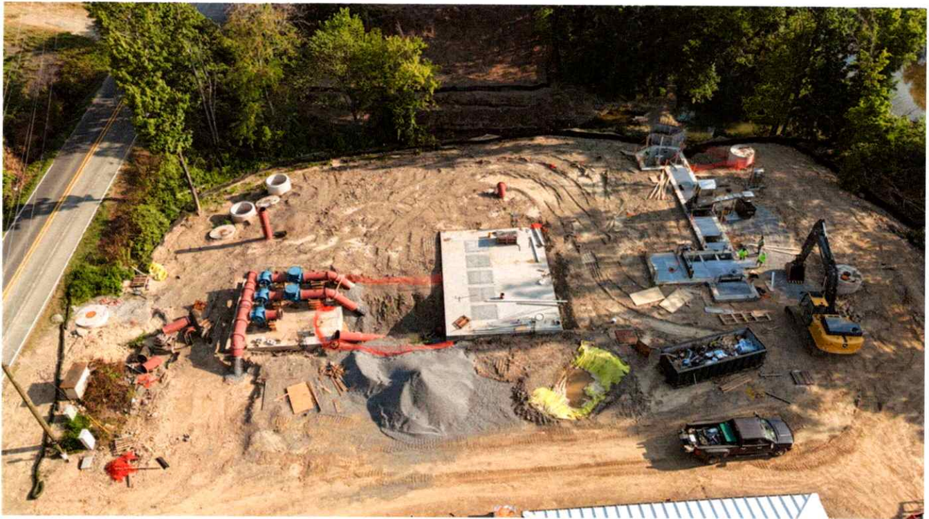
Gulpha Pump Station Construction
