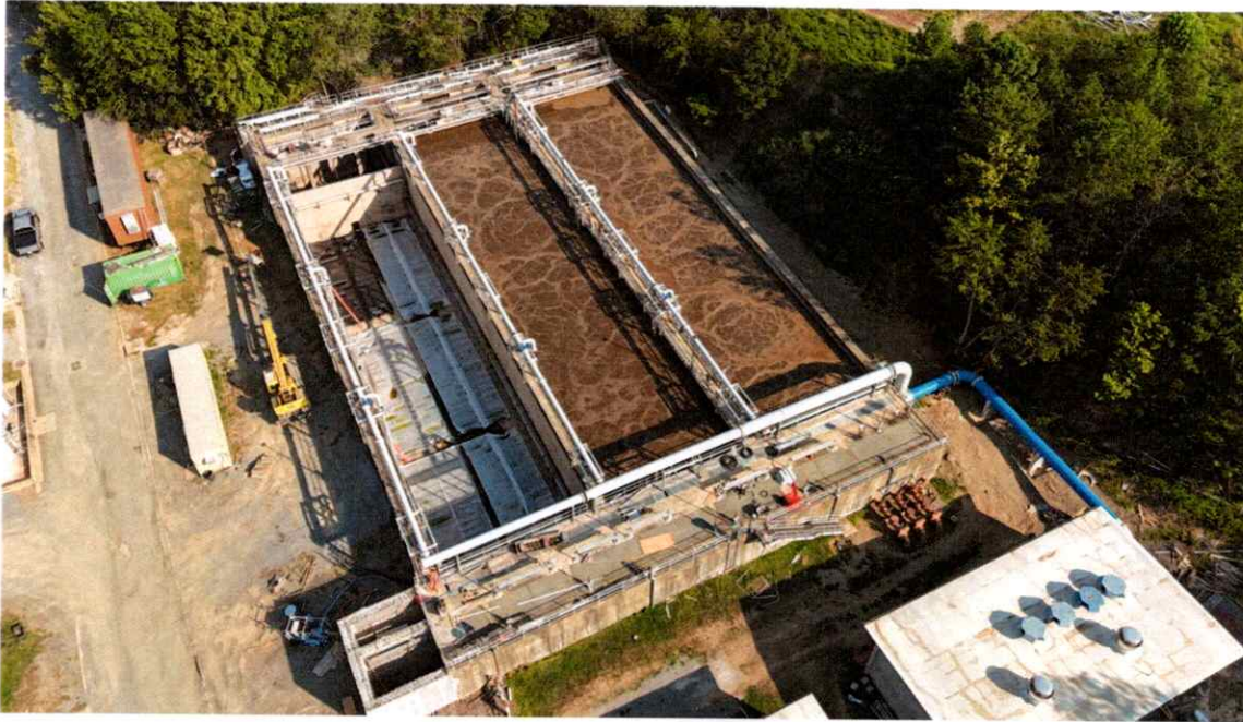
Filter Improvements Under Construction
