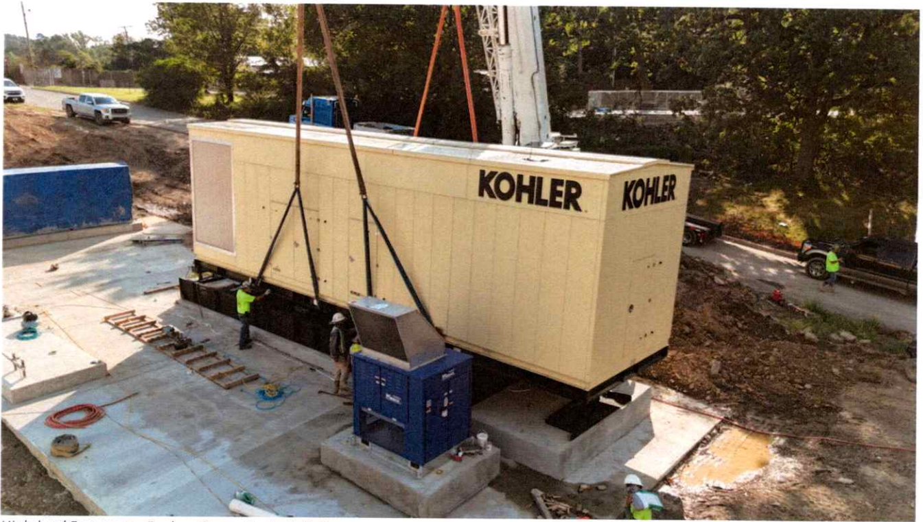
High-load Emergency Backup Generator Installation
